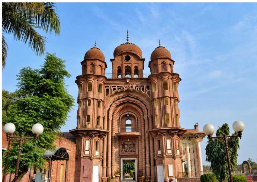
Fig. 8 Principal Entrance Gateway (Front Façade), Gurdwara Rori Sahib (Photo: Muhammad Kashif Ali)
