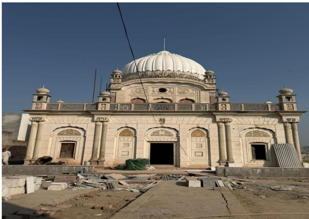
Fig.13 Gurdwara Khara Sahib, under renovation and preservation (Photo: Madiha Abbas)
